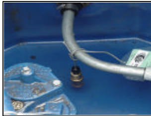
Liquid sump sensor
