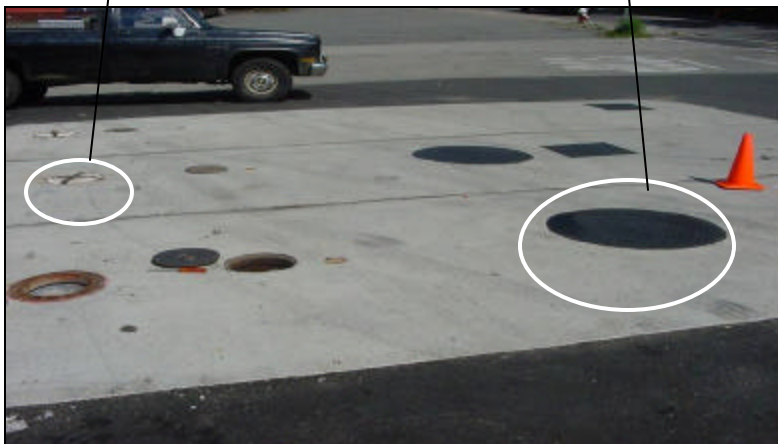
View of sump lids
