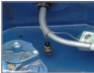
Liquid sump sensor
